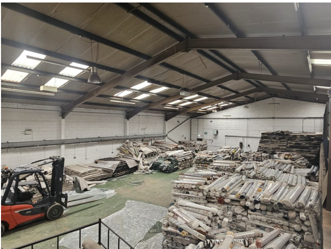
Unit 11 internal from mezzanine
